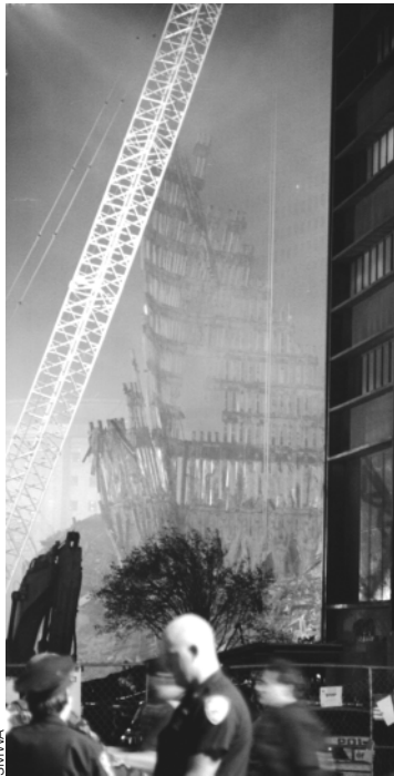
Shell of the tower
